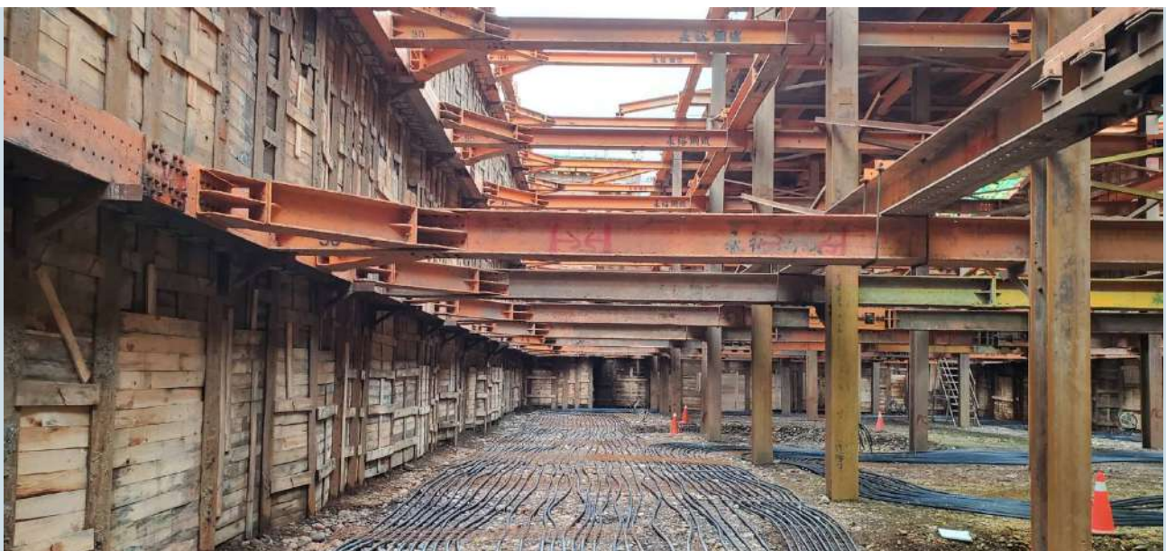
將捷旅閣空調地源管路預埋
